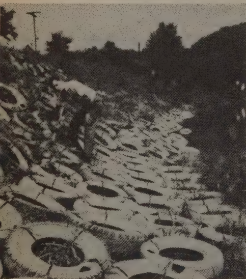
Tire blanket along stream in Little Kanawha, WV.
